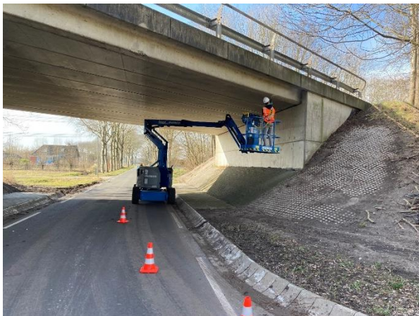
N33: viaduct 07F-314-01.
