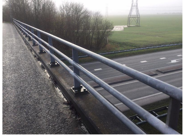
N33: viaduct 07F-105-01.
