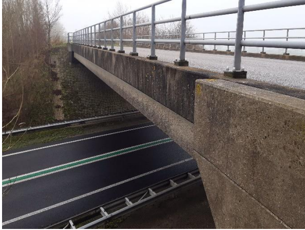
N33: viaduct 07F-104-01.
