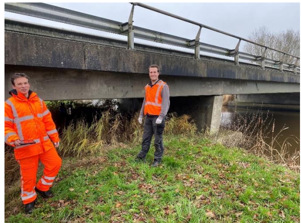
N33: viaduct 07F-313-01.
