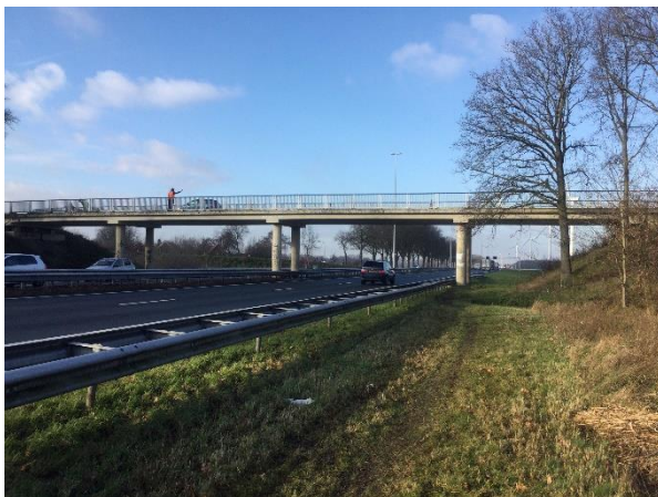
A58: viaduct 1A-104-01.
